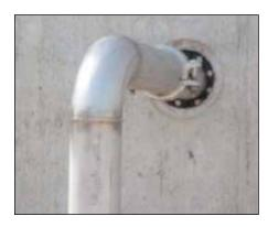
Many of these applications involve connections where the pipe is penetrating a wall, floor or ceiling and sealability is required between the pipe and the penetrated surface. Through wall applications are an area where a mechanical seal needs to be utilized in order to reach complete sealability.
